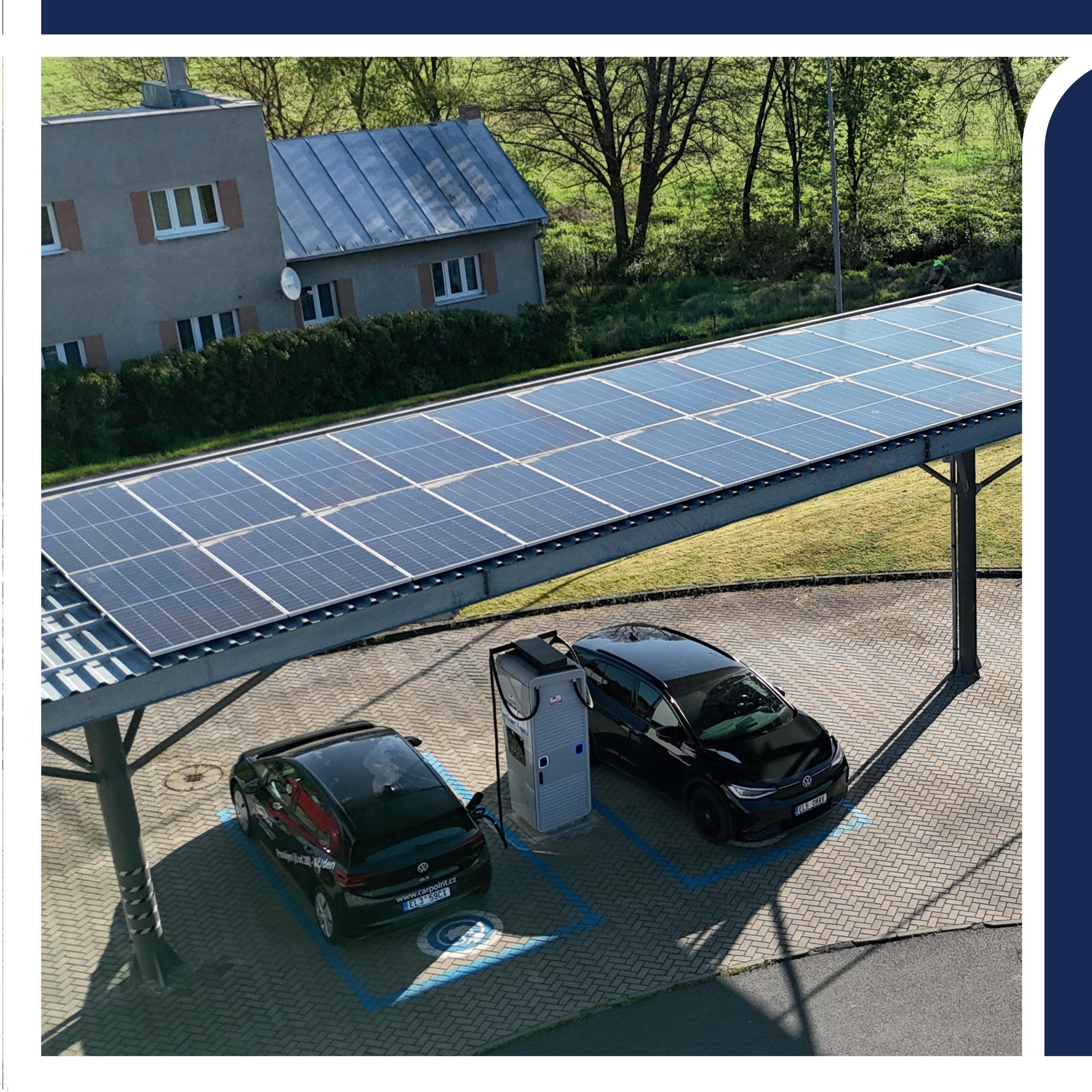
Fast charging station 400kw for e-trucks and e-cars powered by solar and mains current 400V
