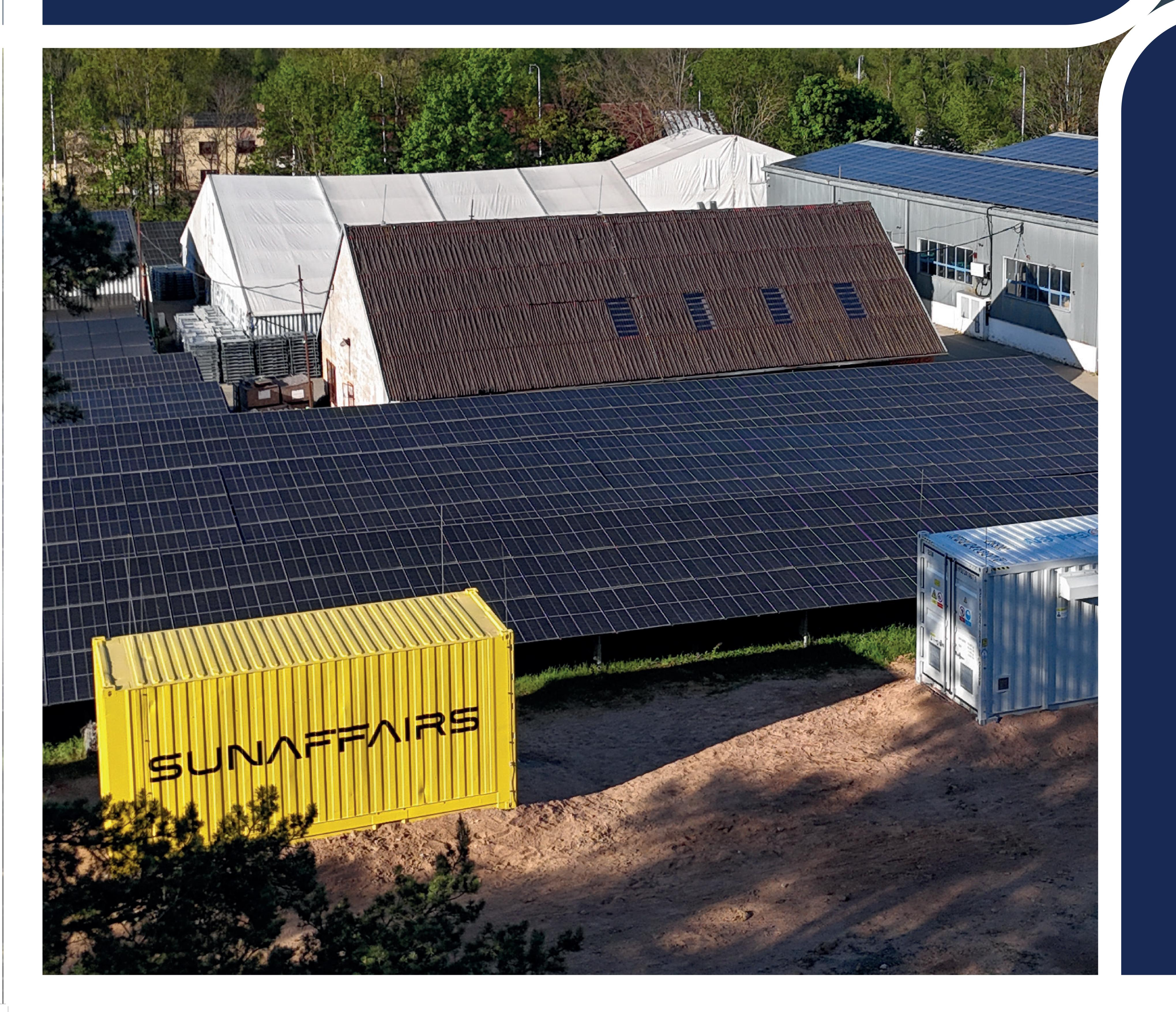
Battery storage 5016kwh with 0.35C maximum charging and discharging capacity
